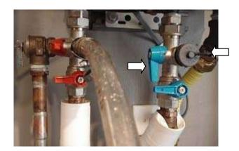
17. Put the hot water drain hose back into the bucket and open the cold water main valve. This procedure will flush out the heater with fresh cold water. Flush for at least 5 minutes or until 20 gallons of water has passed through the heater
