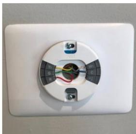
Thermostat Wires - connect thermostat to the furnace
