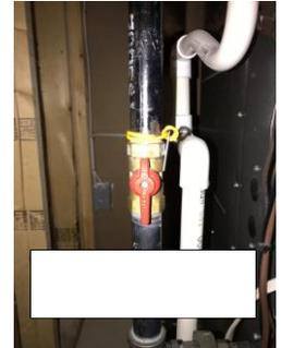
**ELECTRIC FURNACES**: heat will turn off with a clogged condensate drain (the white pipe besides the furnace). Snake out any obstruction to the drain and clean yearly with pouring bleach down the line.
